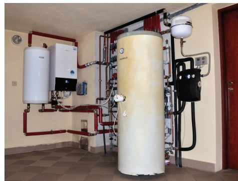
FIGURE 6. Installation of a heat pump cooperating with solar collectors
